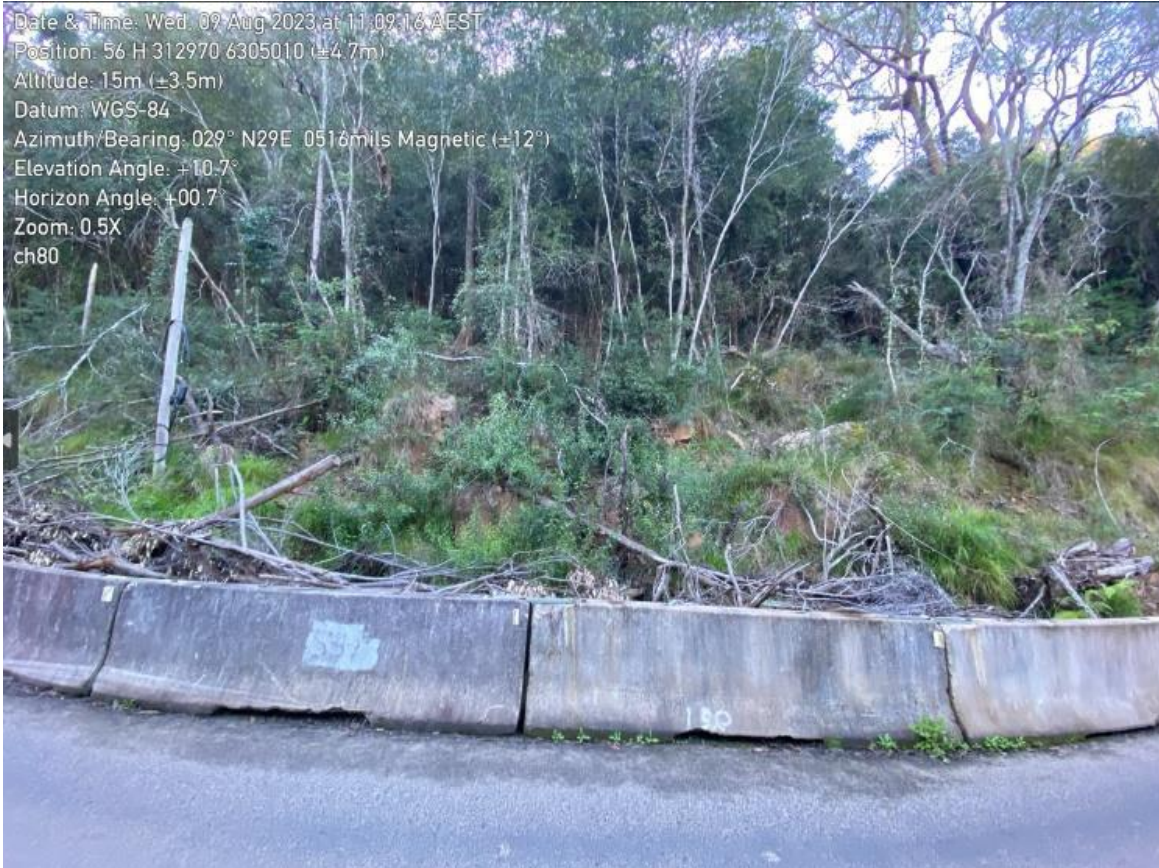
Figure 3-2 views of the landslide looking north east
